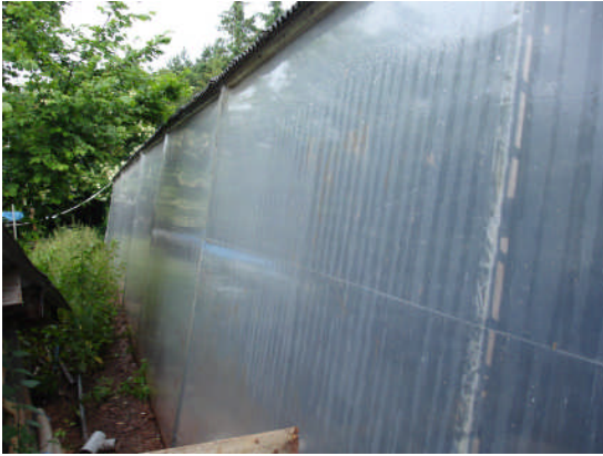
Figure 1 Insulation of Farm Building
